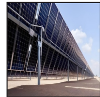
Solar Steel Structure
