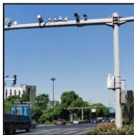
Street Light & CCTV Poles
